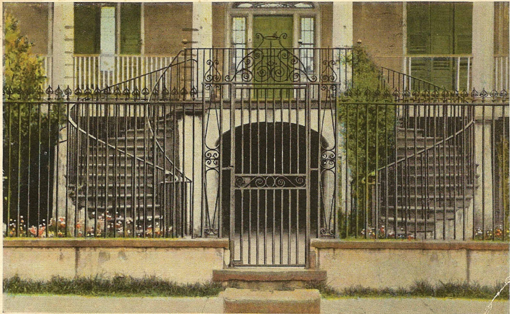
DOOR AND STAIRWAY AT 28 CHAPEL STREET.
